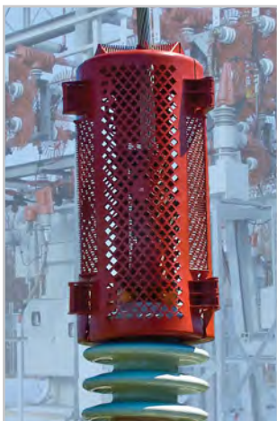
BCAC-IC-8D/18 Bushing Cover
